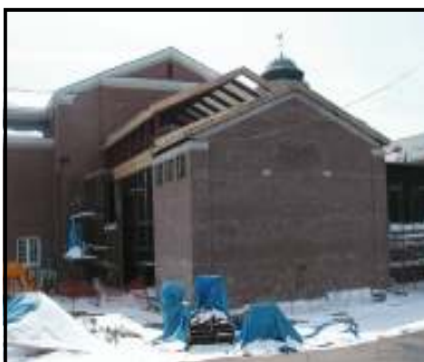
Brick and stone work completed on part of the north elevation
