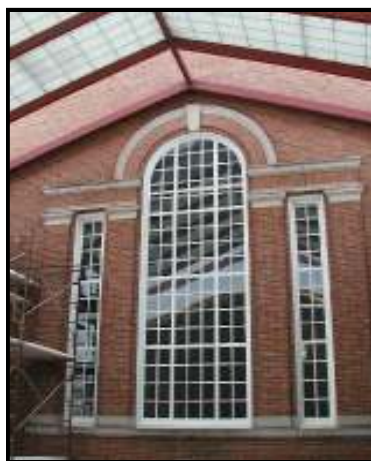
The translucent ceiling in the new entry above the north window
